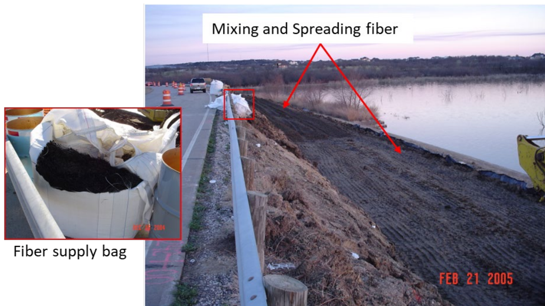
Figure 1.1 Mixing and spreading fiber with soil in PGBT highway project (modified from Gregory 2006).
